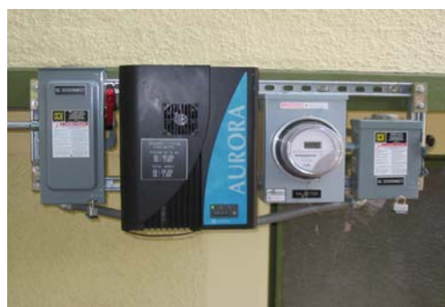
Meter and inverter box
