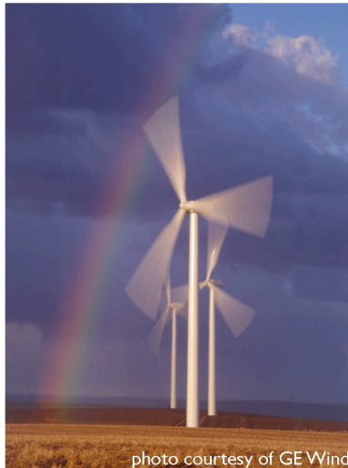
photo courtesy of GE Wind
